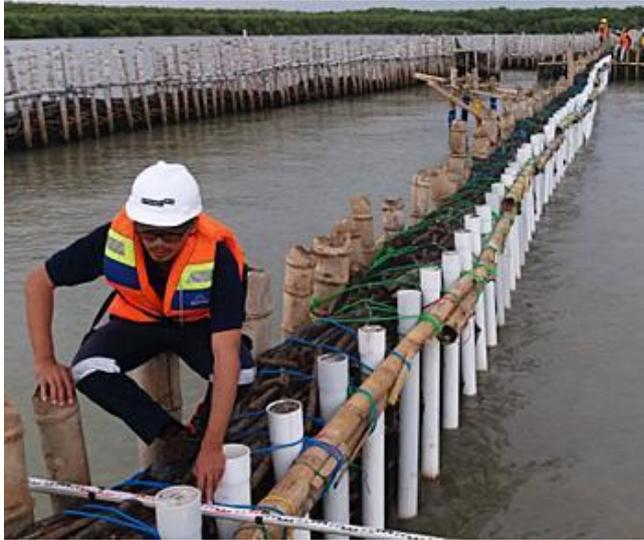
*Figure 6.1 Impression of design (Source: Dutchwatersector, 2018)*
