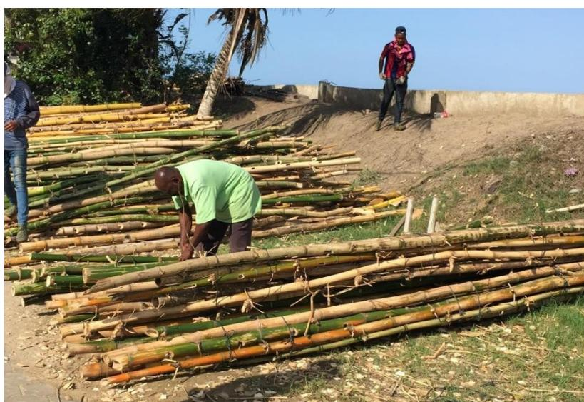
Figure 7.1 Bamboo being prepared for use in the Sediment Trapping Units at the WnZ coast (Source: Ma-Ajong, 2017)
