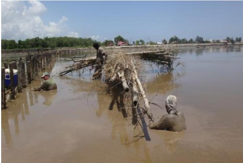
*Figure 6.12 Placing the filling material between the walaba poles (Source: Naipal, 2015)*
